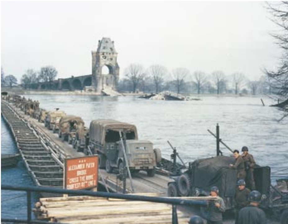
CROSSING THE RHINE. After landing at Normandy, Allied forces liberated France and prepared to move into Germany. Makeshift bridges enabled the Allies to cross the Rhine in some areas and advance deeper into Germany. Units of the 7th U.S. Army of General Patch are shown here crossing the Rhine at Worms on a pontoon bridge constructed by battalions of engineers alongside the ruins of the old bridge.
